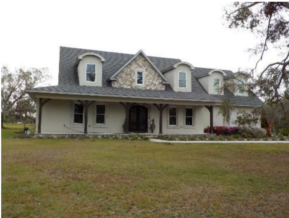
Photograph 1: Front Elevation (West-facing)
