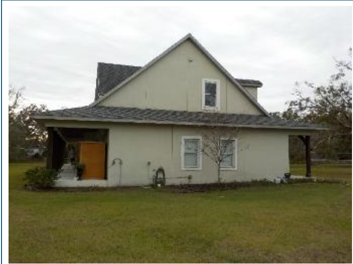
Photograph 4: Left (north) elevation
